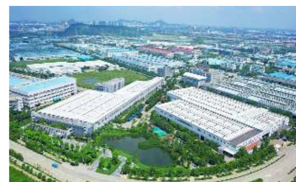
China Gaoli Headquarter and Factory
