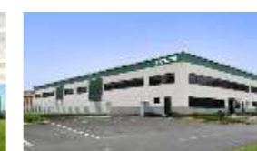
Brazil Joinville Technical Center
